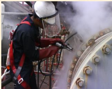
Large flange connection
