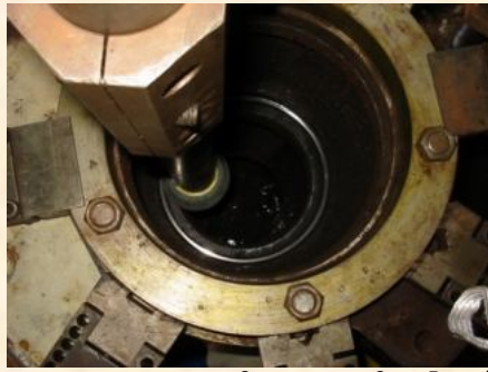
Compressor Seat Repair
